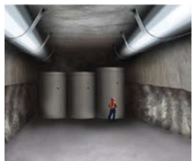
3: Resin Liner Shields within ILW emplacement room
