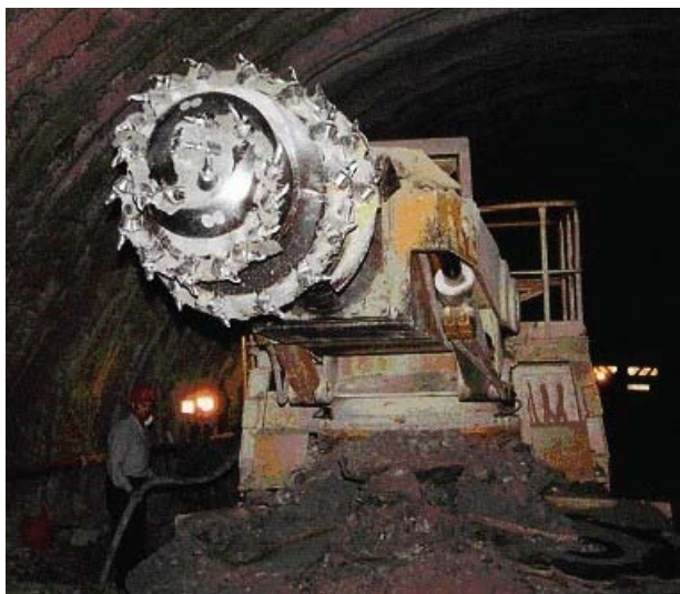
Roadheaders will be used to construct access tunnels and emplacement rooms
