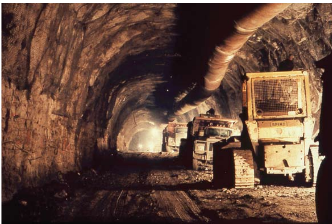
Construction during Darlington cooling water intake tunnel
