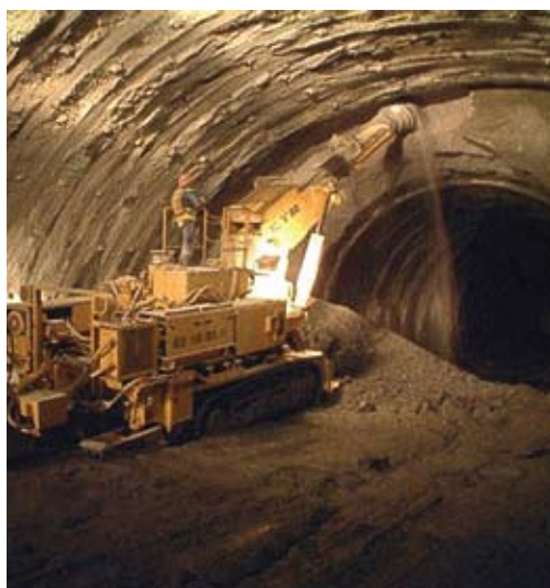
Roadheaders will be used to construct access tunnels and emplacement rooms
